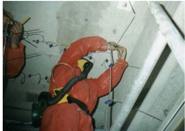
Inserting long needles into sprayed asbestos coating
