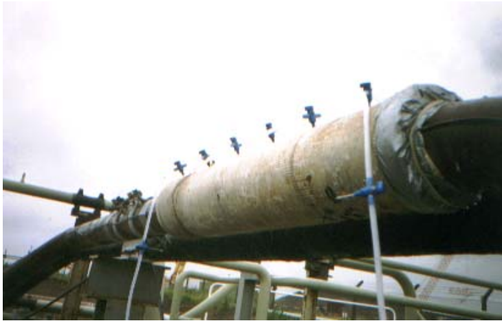
Dust suppression prior to removal by wrap and cut
